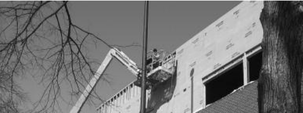
The insulation is put in place front of the building
